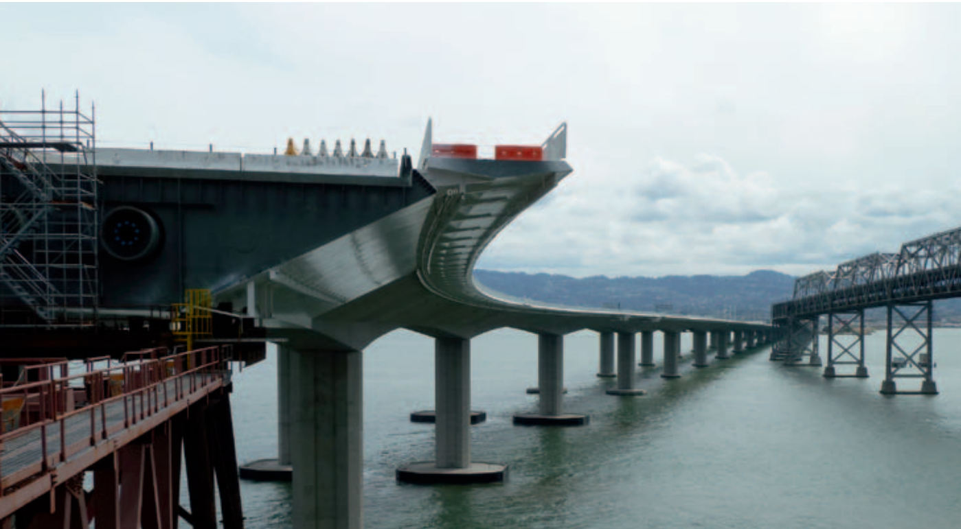
New Oakland Bay Bridge, Muehlhan Certified Coatings
