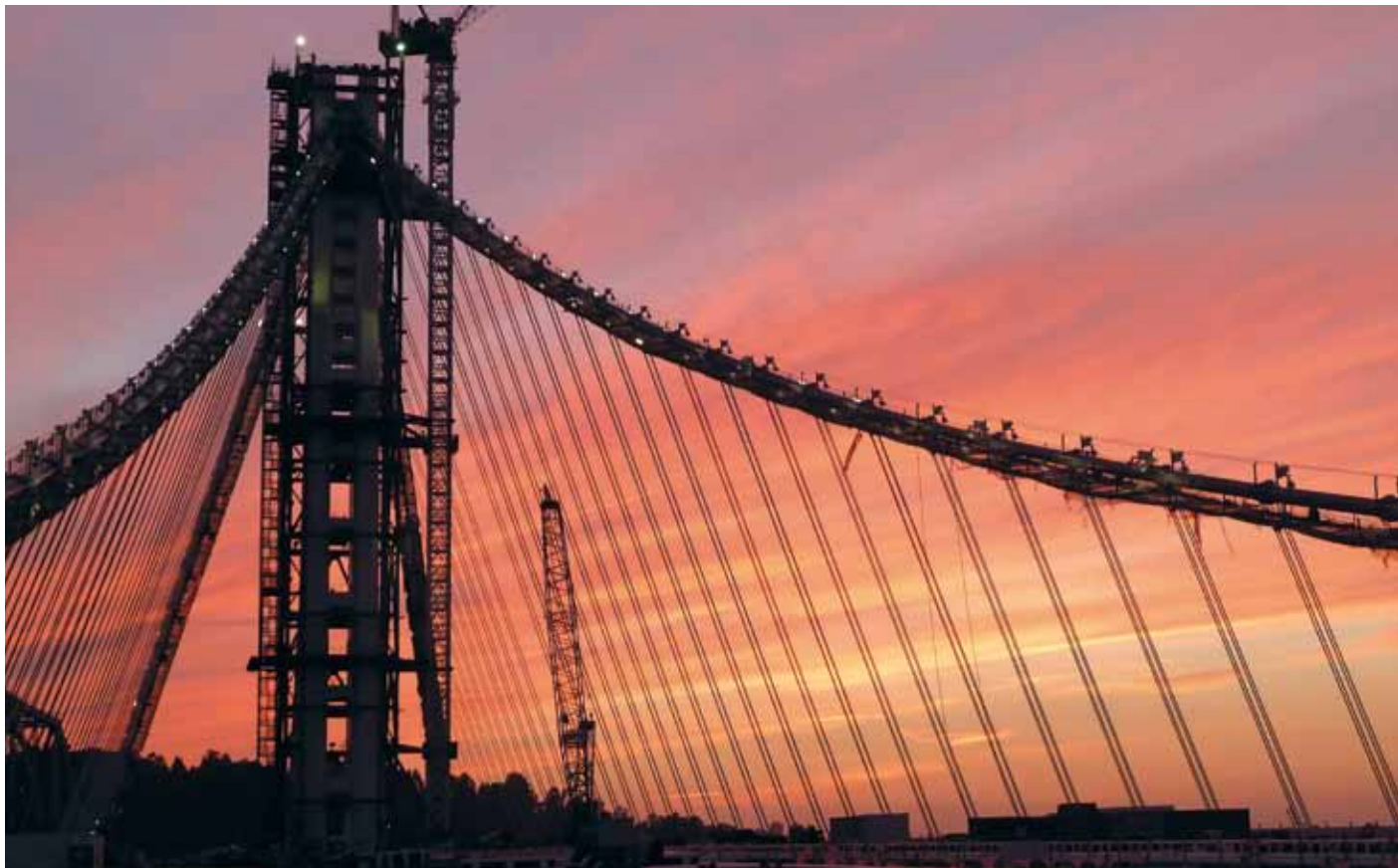
Oakland Bay Bridge, San Francisco
