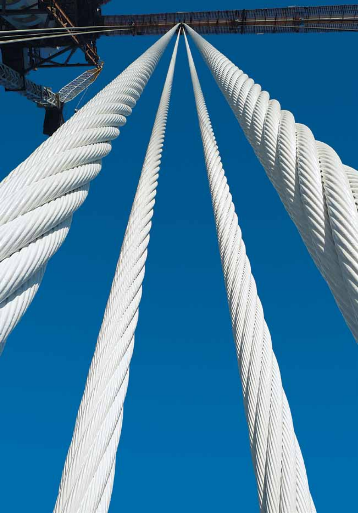
Oakland Bay Bridge, San Francisco
