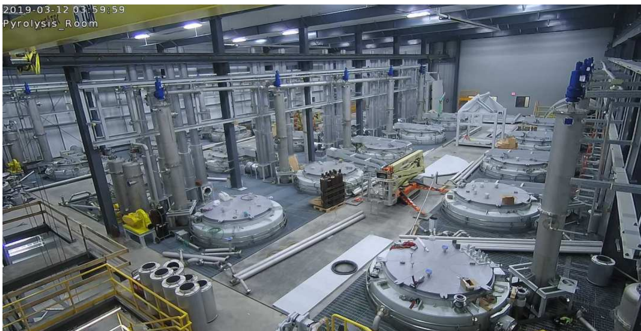
The Pyrolyx production facility under construction in progress in Terre Haute, Indiana (USA) March 2019
