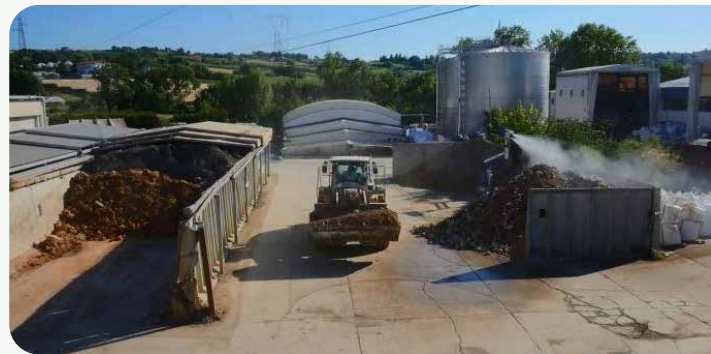
Recycling plant at Rovereta (Rimini, Italy).
