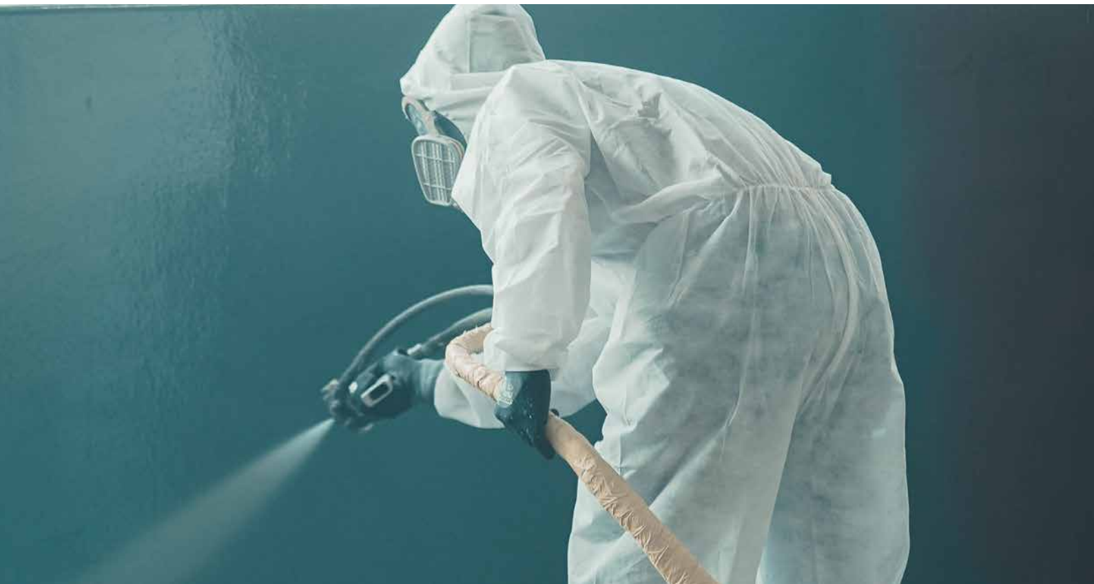
Aboveground tank coating application.
